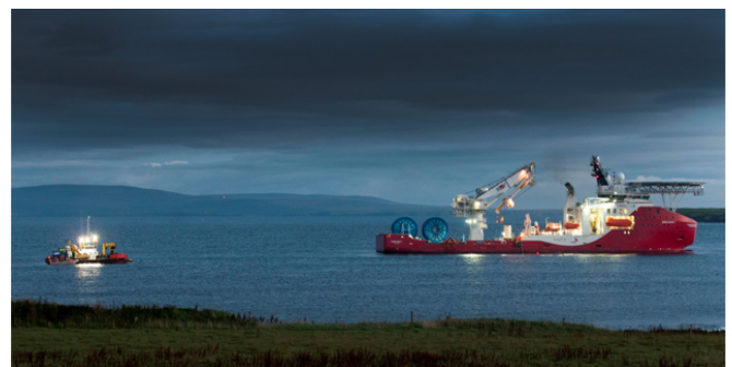
Figure 4 – Export cable installation 2015
