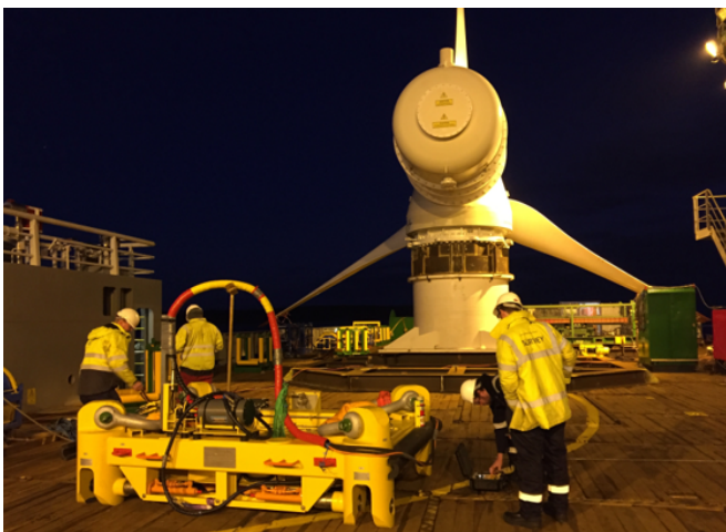
Figure 6 – AR1500 installation with minimal deck spread
