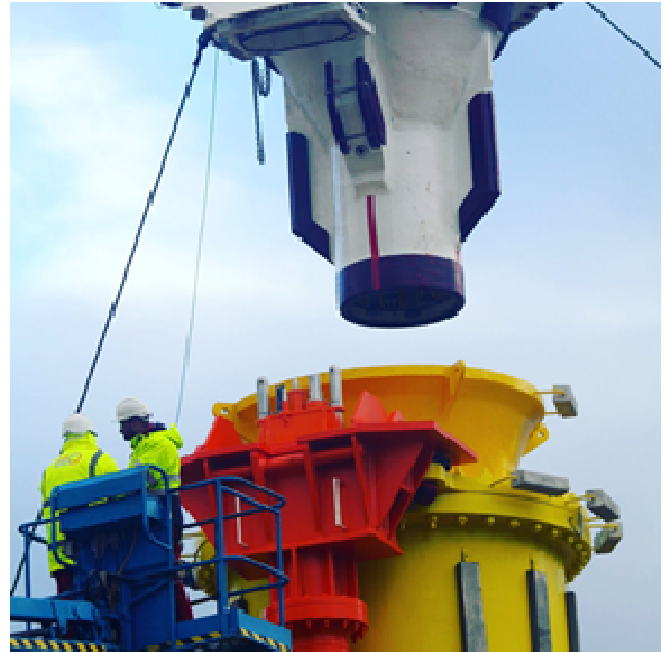
Figure 9 - ARL1500 mating operation (onshore trial)
